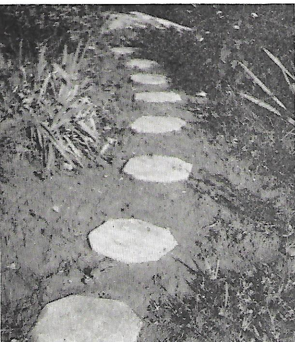
Closeup of octagonal stepping stones which are easily moved from place to place as desired. The richness of the cement mixture coupled with slow drying, makes a durable product of little thickness, giving a stone easily carried about the garden.
