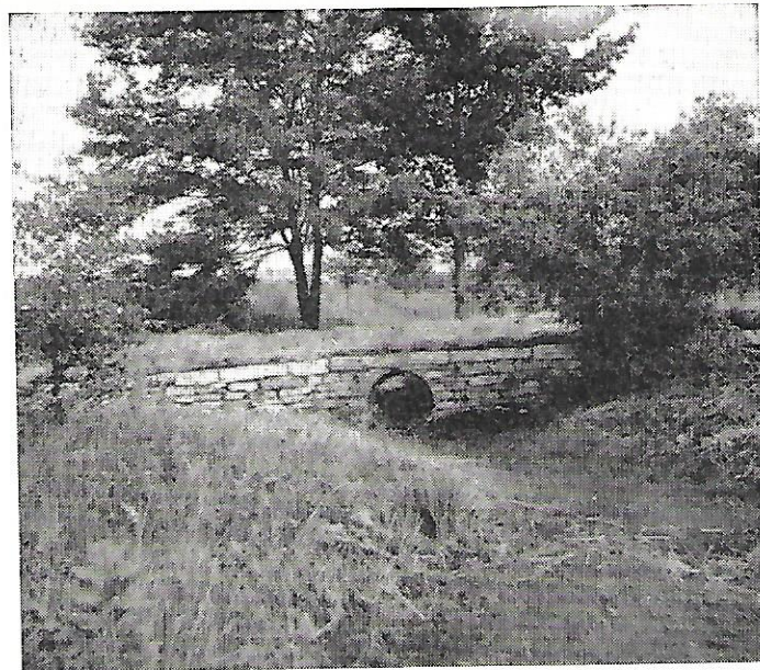
One of the lovely "sod bridges" along the roadside trail at the Lincoln Memorial Garden. These little bridges over small ravines offer great possibilities for effective planting.
